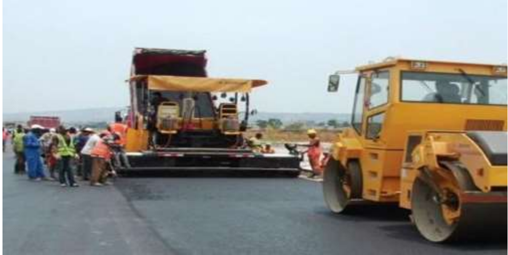
Figure 2.8: Muritala Muhammed airport Road's Reconstruction
