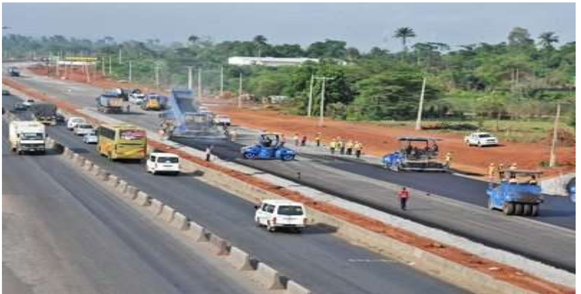
Figure 2.9: Reconstruction of Lagos-Ibadan expressway
