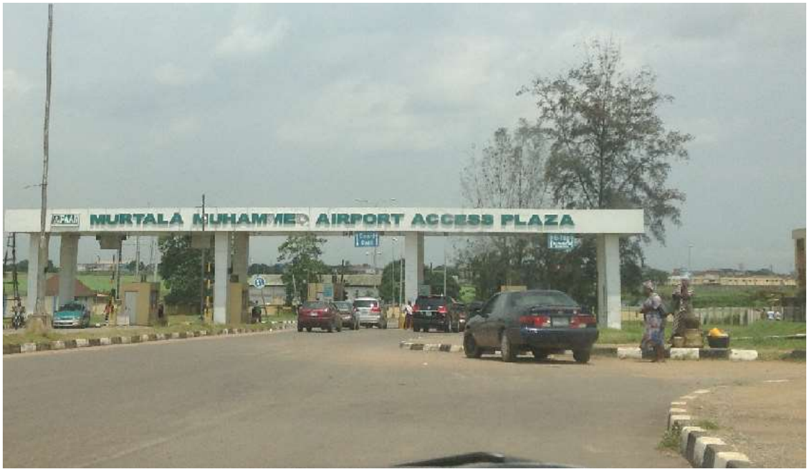
Figure 2.7: Muritala Muhammed Toll road
